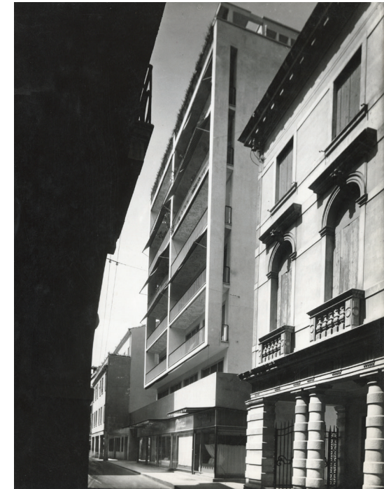
Fig. 1 - The First IRE Building. Historical photograph (Archivio del '900, Man.-Mio.3.3.46.1.1.9).
