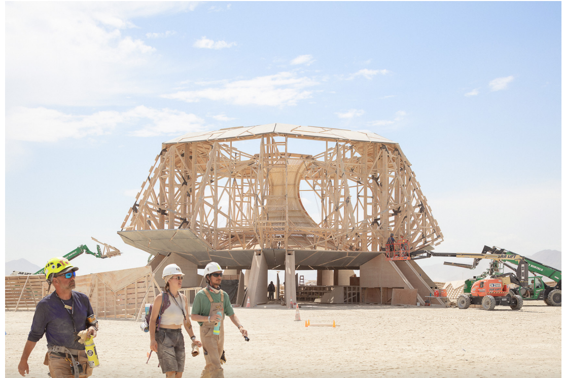
Figure17. Burning man temple construction. Photograph by Milena Villalba
