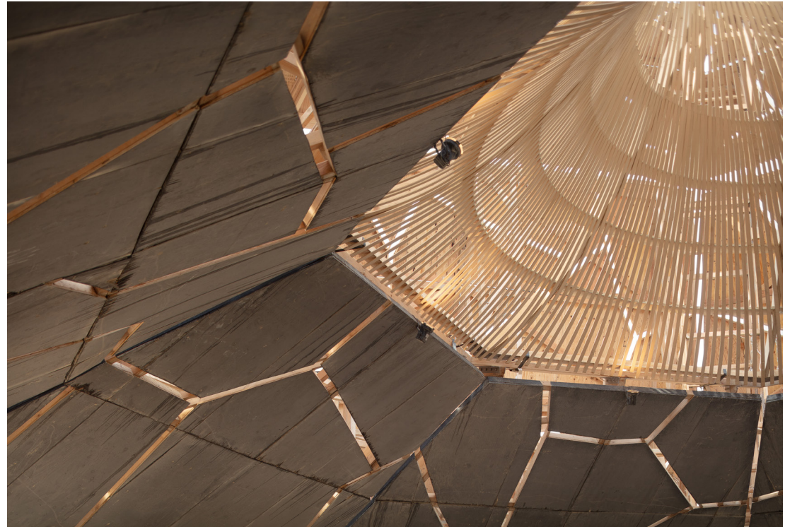
Figure18. Façade detail. Photograph by Milena Villalba
