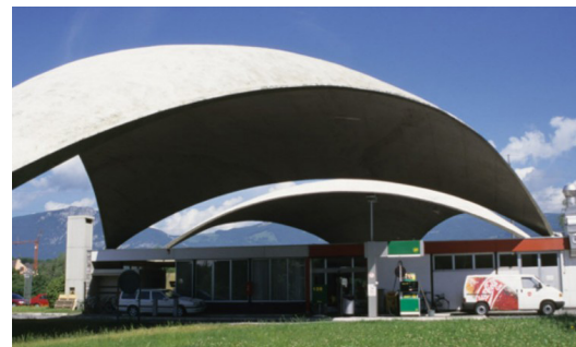
Fig. 7. H. Isler, Roof structure of Deitingen Süd Service Station, Switzerland.
