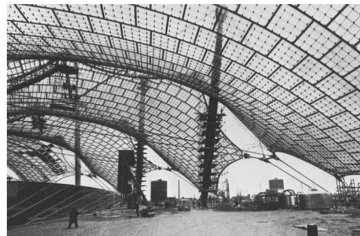
Fig. 5. F. Otto, Roof structure of the Munich Olympic Stadium.
