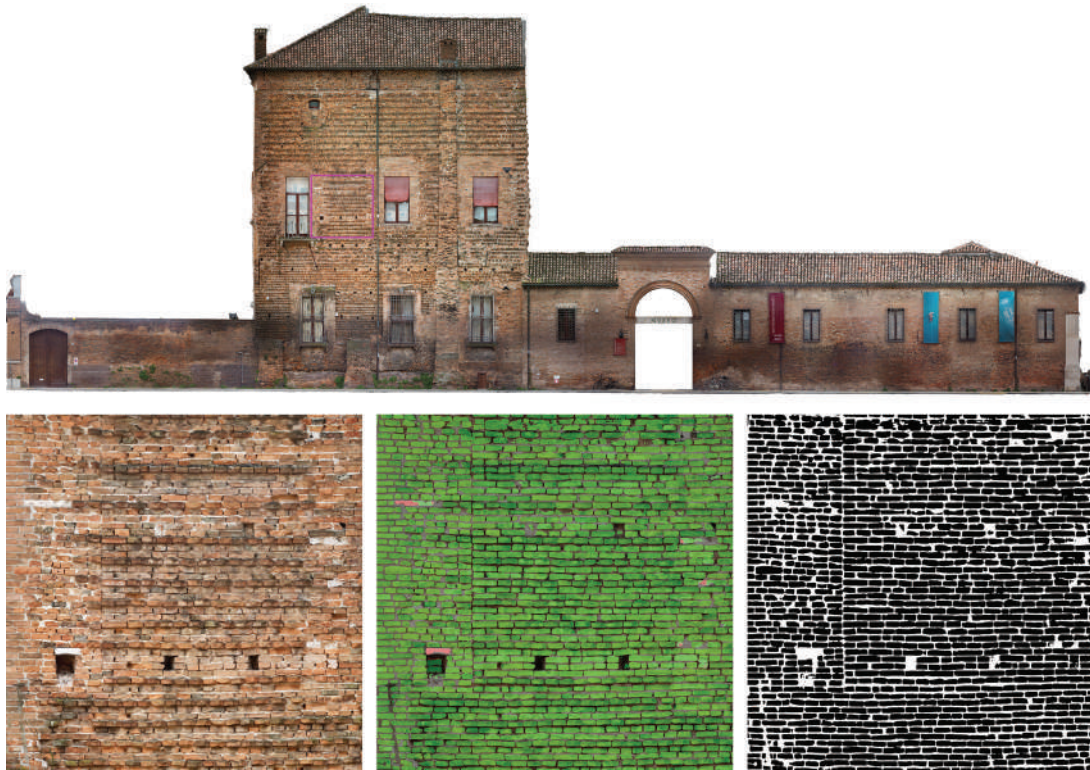
Figure 10. Analysis of a portion of the masonry of the main façade. Morphologically complex elements, such as variations in the plane or sawtooth patterns, are not captured by the automatic segmentation. Graphic elaboration by the authors.
