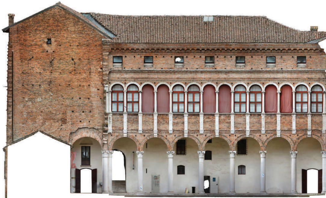
Figure 4. West Elevation of Cortile d'Onore , orthomosaic obtained from photogrammetric processing. Graphic elaboration by the authors.
