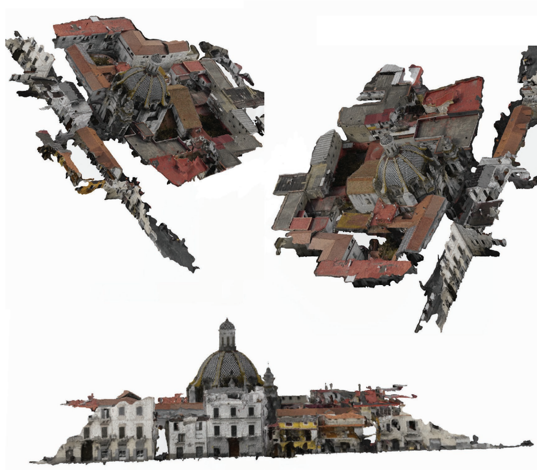
Fig. 6 - Views of the 3D model from the drone survey. Survey by Mario Ronca, supervisor Manuela Piscitelli.
