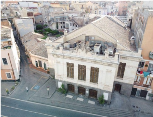
Fig. 6 - Top view of Teatro Bellini in Adrano taken by drone.
