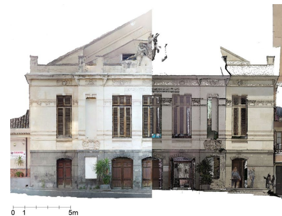
Fig. 10 - Orthophoto of the main façade of the Teatro Massimo Bellini in Adrano. On the left, UAV point cloud, on the right, TLS point cloud.
