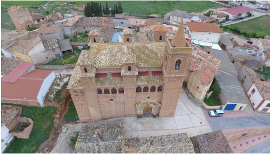
Fig. 3 - Photograph taken with an unmanned aerial vehicle (UAV) of the exterior of the Church of San Félix (Torralba de Ribota).
