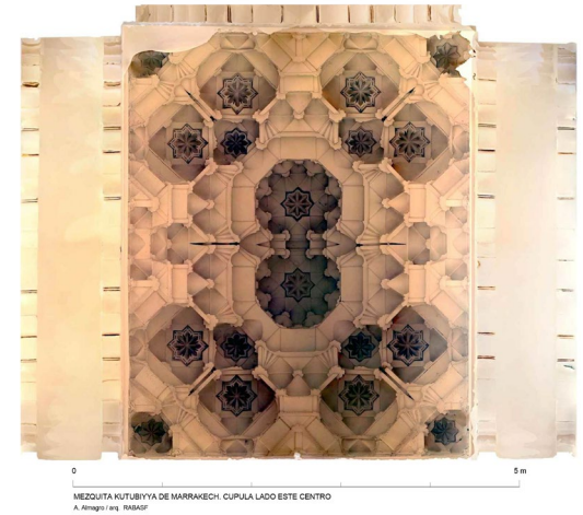
Fig. 3 - Orthoimage to scale of a muqarnas vault from the Kutubiyya mosque in Marrakech
