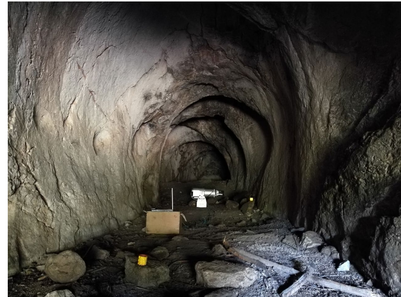
Fig. 4 - Scanning activities of the southern portion of the tunnel.
