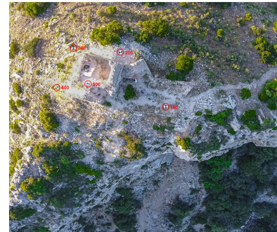
Fig. 7 – Aerial view of the tower. The targets situated at the TS points are on the ground.
