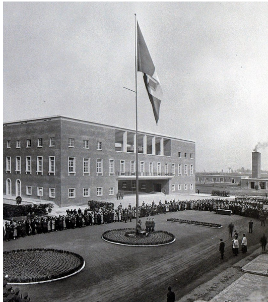
Fig. 5 - Grand opening of the architectural complex
