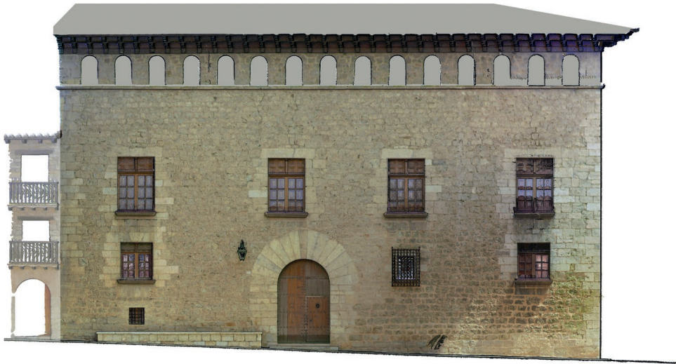
Figure 8. Image obtained from the point cloud of the building's façade. 2023
