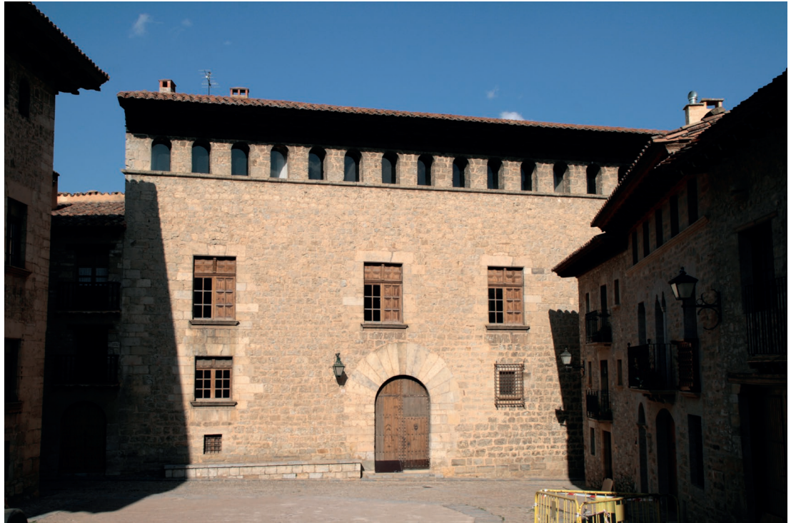
Figure 7. View of the south façade of the Casa Castellot. 2023
