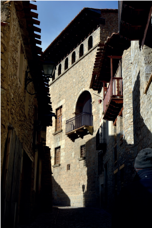
Figure 6. View of the west façade of the Casa Castellot, overlooking the Plaza Aliaga. 2023
