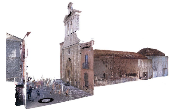
Fig.6. Laser scanning of the chapel of San Ildefonso showing the complete architectural organism treated. By the authors.
