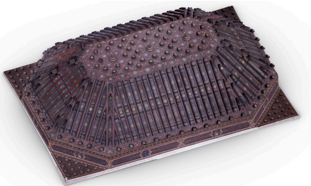
Fig.15. Photogrammetric model of the Coffered ceiling of the head of the chapel of San Ildefonso. By the authors.
