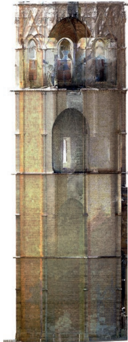
Fig. 1 - Ortophoto of the "Miguelete" Bell Tower of Valencia Cathedral, captured using a laser scanner.
