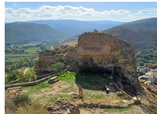
Fig. 3. General view of the north wall of the castle of Ademuz.
