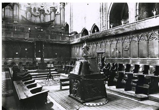
Fig. 1 - Condition of the original masonry. (CRDI Girona City Council)
