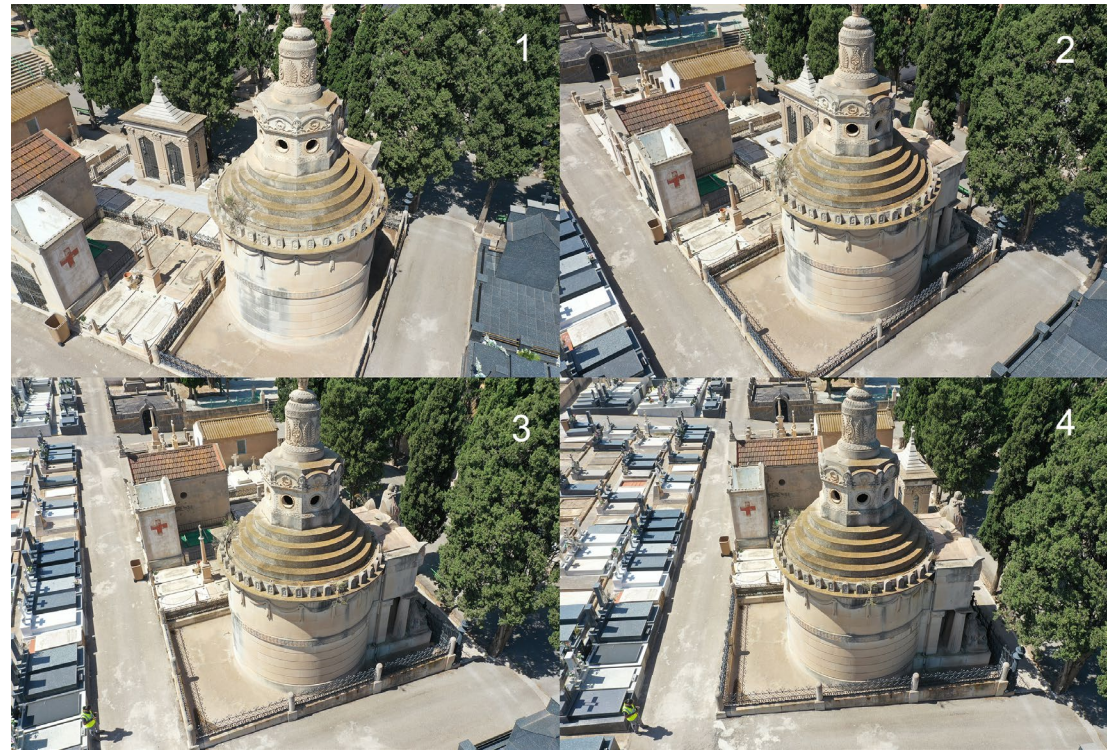
Fig. 4 - Sequence of 4 concentric aerial frames taken with the RPA to define the stepped dome and lantern of the pantheon. Authors
