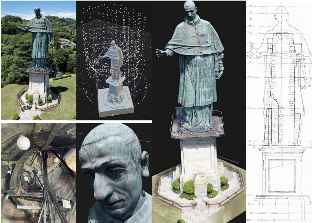
Figure 2. The Colossus of San Carlo Borromeo in Arona (NO). Top: DJI Air2s drone survey of the exterior of the statue for high-resolution orthophotos (3D photogrammetric model prof. Luigi Barazzetti); bottom, Faro CAM 2 Focus laser scanner survey of the interior of the head. Right, vertical section in scale 1:25 from 1974, made by engineer Carlo Ferrari da Passano (source: Veneranda Biblioteca Ambrosiana Archives). The purpose of the 1:20/1:10 scale 3D detail survey was the structural consolidation of the internal metal anchors of the statue's copper plates.
