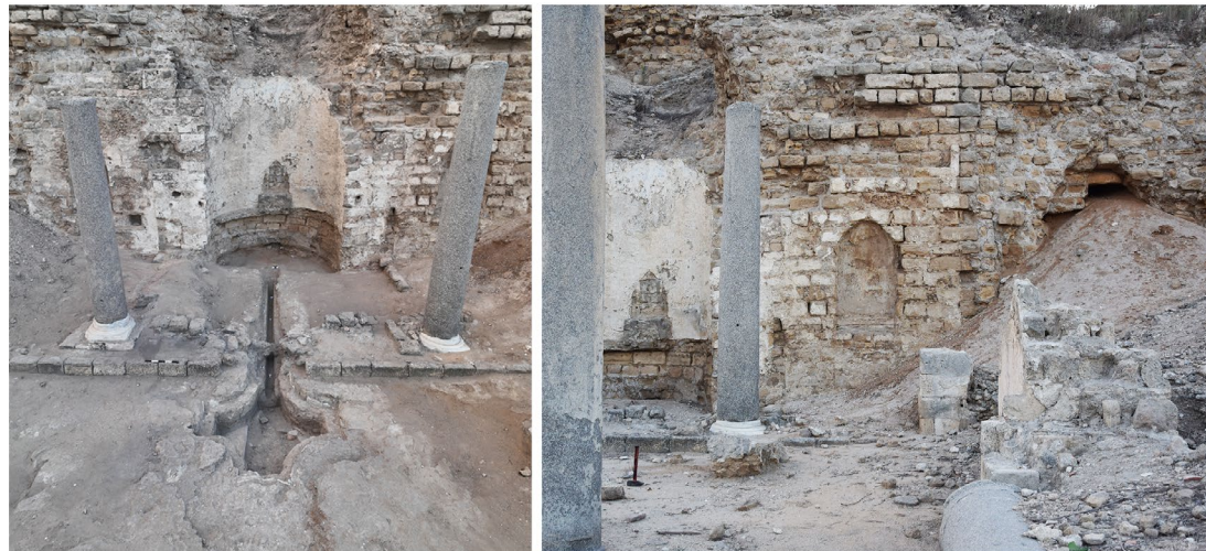
Figure 2. Detail images of Santa Maria in Viridis: on the left, the water channelling system from the apse to the cruciform font; on the right, one of the niches flanking the apse.
