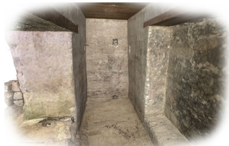
6J2-Sub2 Building + Structure 1 Interior
