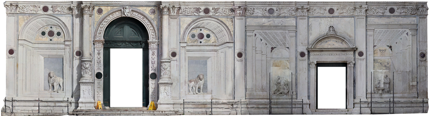
Fig. 4 - Lower register of facade taken from the orthorectified image of the School.
