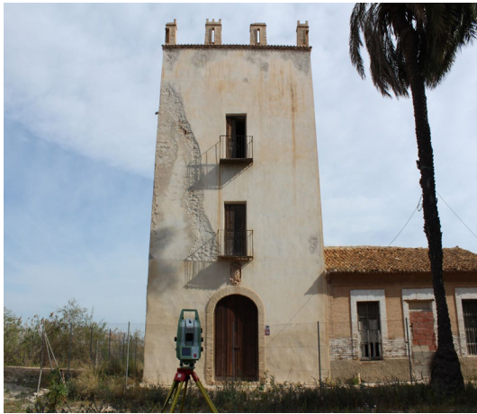
Figure 6. Data capture of the Rame tower.
