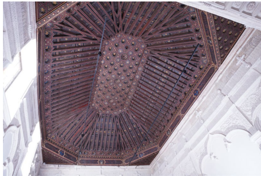
Fig. 6 - Wooden coffered ceiling. San Ildefonso Chapel. Photography and 3D printed model. By the authors
