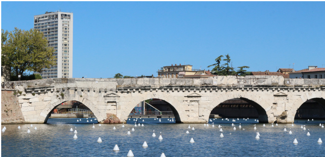
Figure 1 - Tiberius Bridge in Rimini, south elevation. Photo by the authors.
