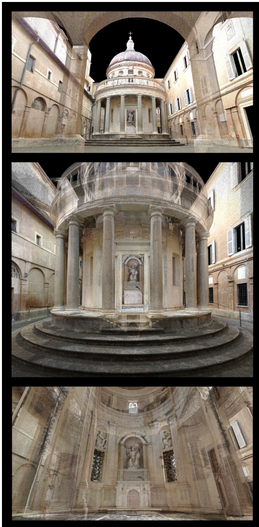
Fig. 4 - Numerical model obtained by laser scanner. Starting from the top: image taken from the porch inside the courtyard, image taken near the colonnade, interior image of the naos environment.
