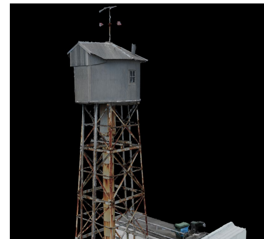
Fig. 3 - Colonial Ammunition Shot Tower. Rendered Photogrammetry Mesh – Credit Sam Smith and Maksym Khovalko, model based on drone recording by Regan Potangaroa and Renata Jadresin-Milic, 2023
