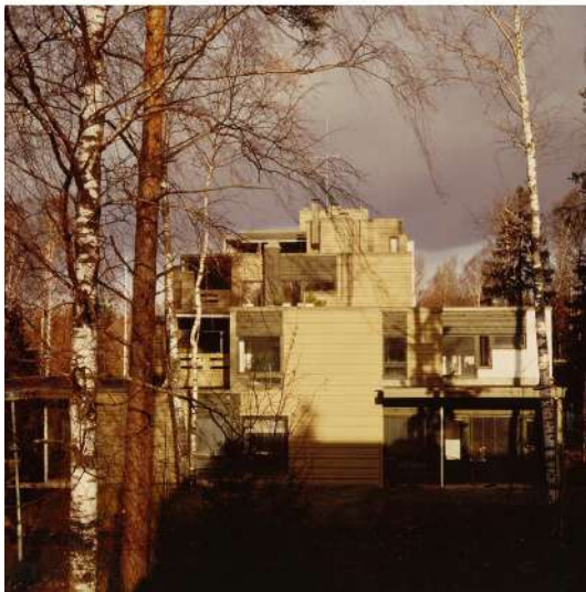
Fig. 19 - Photographs of the Suvituuli building, ca. 1984 (source: the MFA).
