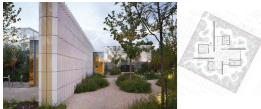
Fig. 17 - Photograph and plan of Maggie's Southampton Centre by AL_A. Photograph by Hufton+Crow. Source: AL_A
