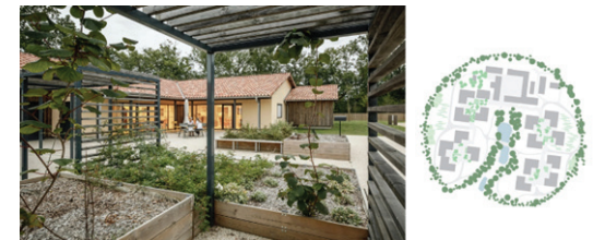
Fig. 15 - Photograph and plan of Le Village Landais Alzheimer in Dax by NORD Architects. By 11h45. Source: 11h45.
