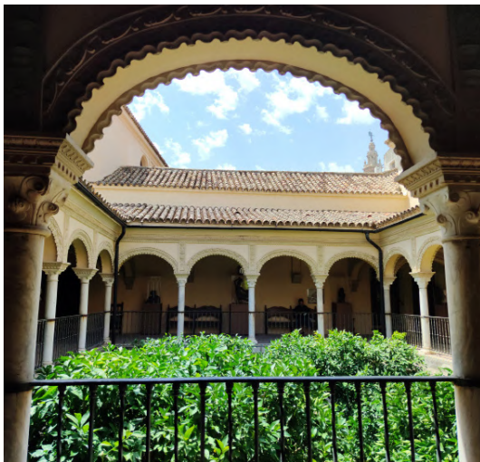
Fig. 11. High gallery at the main patio with recovered arches without plaster decoration and current state. Source: Rafael Manzano archive (RMM), 1970; Own photograph, 2025.
