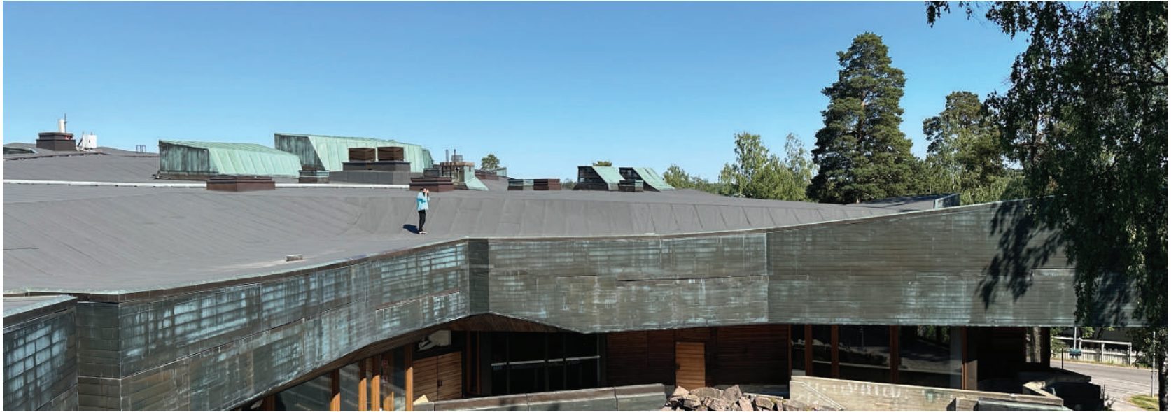
Fig. 20 - Photograph of the visit to the Dipoli roof (the author' photo, 2024).
