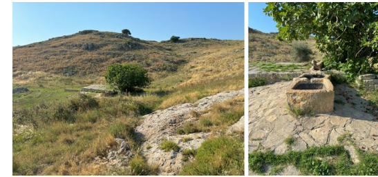
Fig. 18- Caption of the figure 18, Stone channels to collect water from the slopes of the hills in the Jazzo Da Figlia, in the background the buried cistern and watering hole for the animals to drink the collected water. Photograph by the authors.
