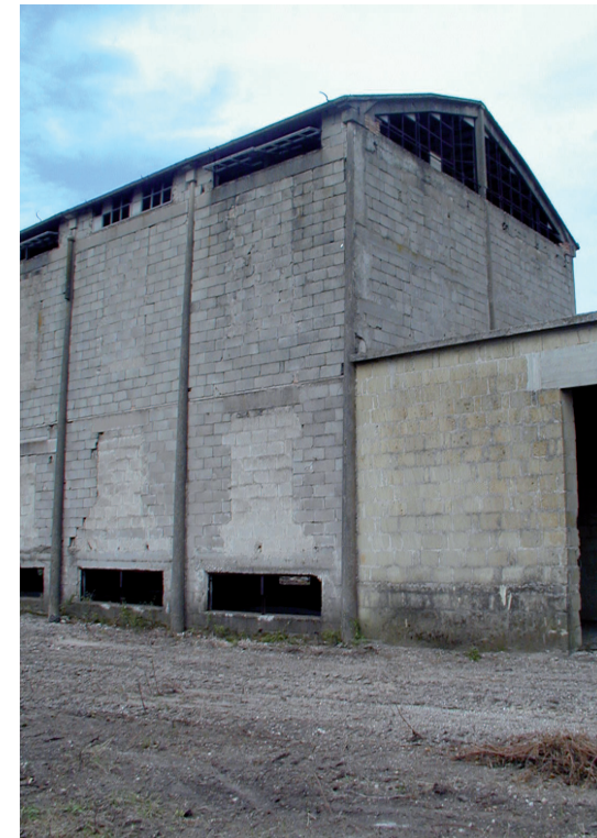
Fig.07 - Tobacco Factory in Presenzano: drying room (photo by the Authors).
