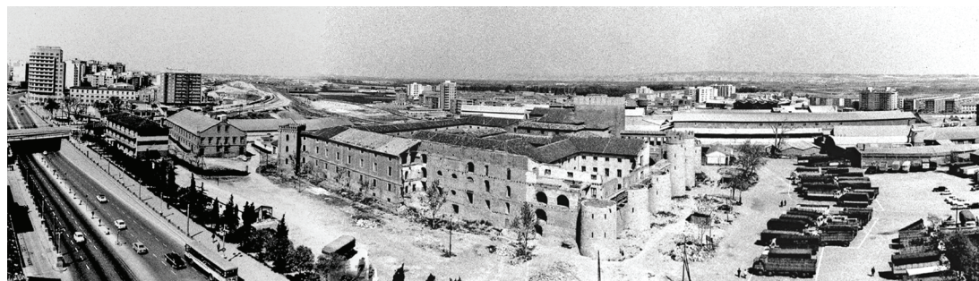
Fig. 9 - Panoramic view SE during the demolition of the barracks in 1973. Photograph: Gerardo Sancho Ramo. Great Archive of Ancient Zaragoza Project (GAZA)
