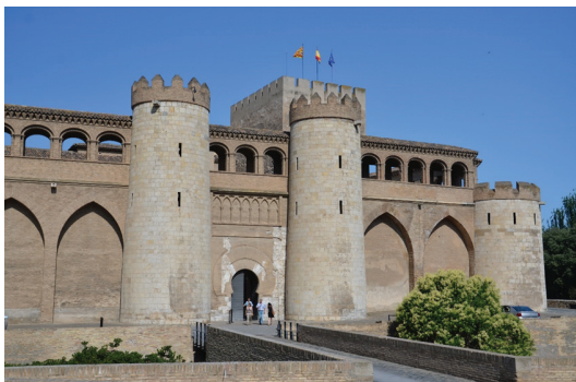
Fig. 6 - View of the main entrance to the Palacio de la Aljafería and the reconstructed bridge. Photograph: E. Bailliet (2012).
