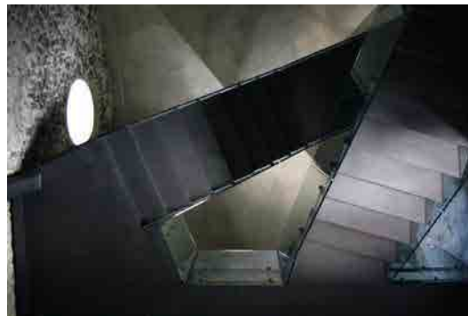
Fig. 1. Bottom view of the steel staircase
