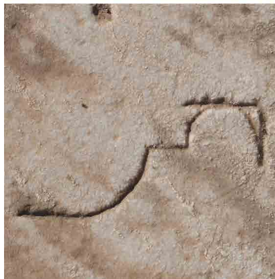
Fig. 1 - Example of worksite tracing. Roman forum, Rome, attic base engraving on stone element; Theatre of Mileto. Molding of the outer closing wall of the cavea; Pergamo, Dioniso's Temple, working tracing for column's bases; Pantheon, Rome, engraved circles for the realization of the drill strings of the pronaos internal pylons.
