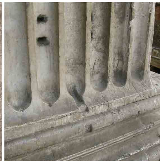
Fig. 1 - Example of worksite tracing. Roman forum, Rome, attic base engraving on stone element; Theatre of Mileto. Molding of the outer closing wall of the cavea; Pergamo, Dioniso's Temple, working tracing for column's bases; Pantheon, Rome, engraved circles for the realization of the drill strings of the pronaos internal pylons.
