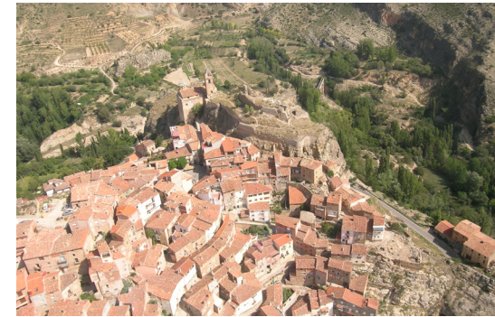
Figure 1. View of the town with the "acropolis" of the castle and the fortress/church over a bend in the river Ebrón.
