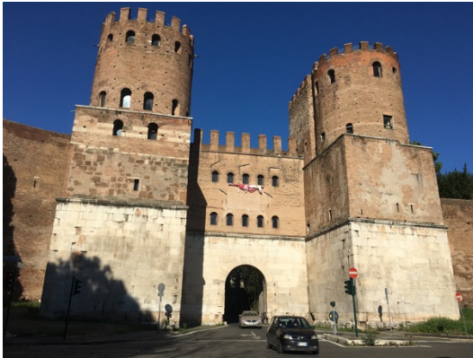
Fig. 6 - "Porta San Sebastiano", venue of the Museum of the Walls.
