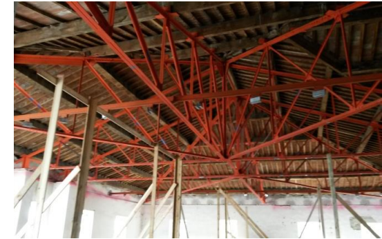
Fig. 19 - "Tobacco Factory" in Arezzo. The roof frame
