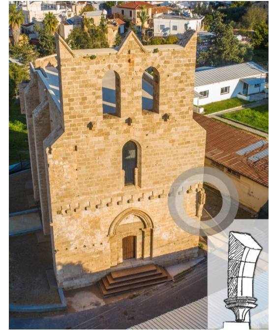
Fig. 7 - Bracket of an octagonal arch. Drone's view of St. Anne and a drawing published by Enlart.
