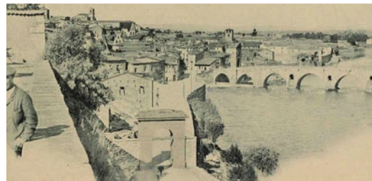
Fig. 8 - Road and "El Pescado" gate, in their original location.
