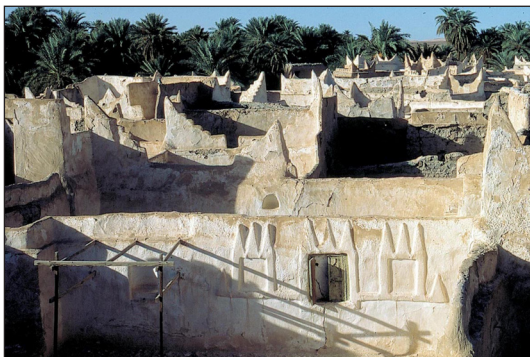
Fig. 19 - Ghadames, the skyline of the serafin in the corners of the buildings' terraces. (Picture by the author, 2004).
