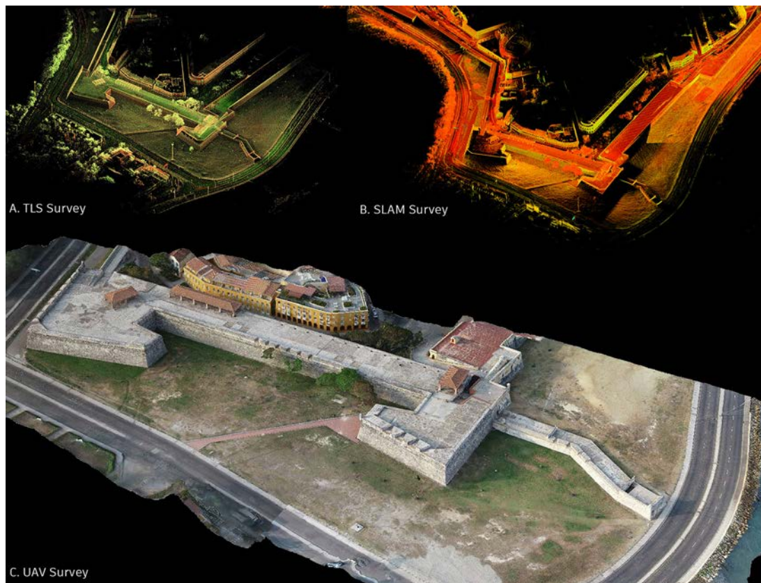
Fig. 13 - St. Catalina and St. Lucas bastions in a comparison of different level of point cloud detail: TLS, SLAM and UAV acquisition.
