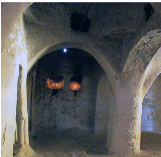
Fig. 8 - Connection between cube and hemisphere in buildings without morpho structural transition elements. Above: the problem of covering the corners of the square. In the middle: a marabout from Matmata, Tunisia. Below: the inner space of the mosque of the Seven Sleepers in Chenini, Tunisia, where the corner covering shelves are evident.
