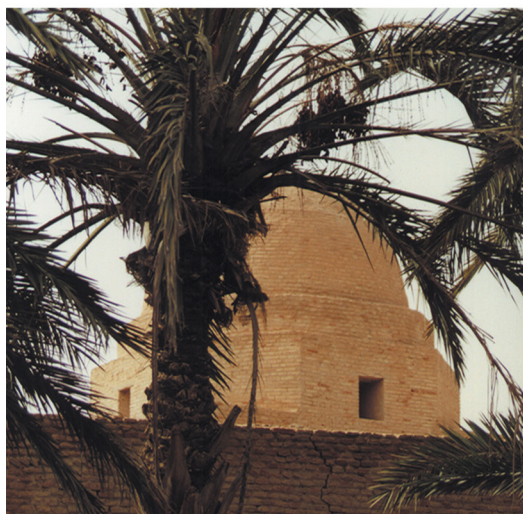
Fig. 9 - From the square to the octagon. Above: a) superposition of two squares; b) octagon deriving from the corner shelves; c) octagonal connection drum; d) progressively cantilevered drums. In the middle, below: two marabouts from Nefta, Tunisia (photo by P. Raffa).
