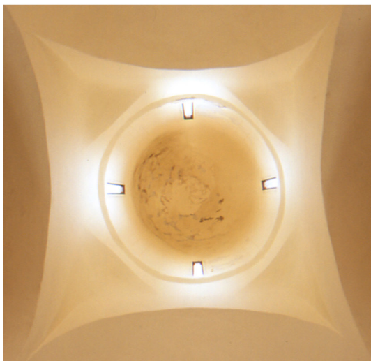
Fig. 12 - Pendentives. Above: dome of the Cattolica in Stilo (Reggio Calabria), 9th-10th century. Below: dome of the church of S. Filomena in Santa Severina (Crotona), 11th century.
