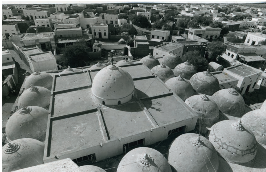
Fig.13 - al-Zaydiyya Mosque. The central part of the building is modern, filling the space of the former courtyard.
