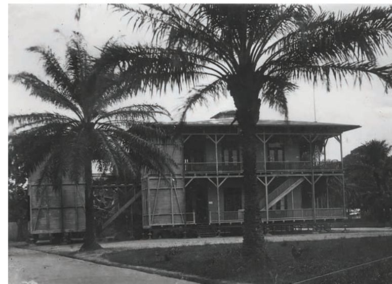
Fig. 11 - Prefabricated house exhibited at the Berlin Colonial Exhibition in 1896, rebuilt in Douala to serve as headquarters of the district offices, 1902 (Stiftung Preußischer Kulturbesitz, VIII A 9200).
