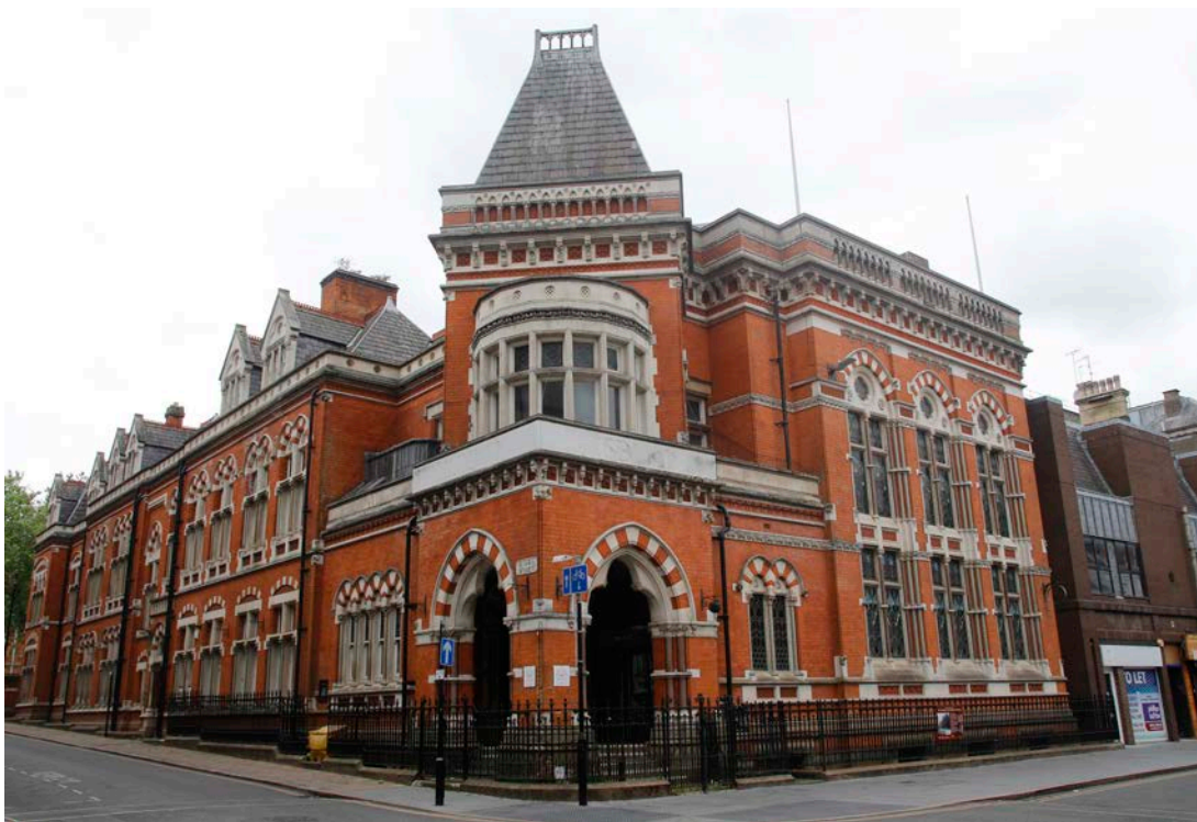
Fig. 18 - The former HSBC building in 2020.
