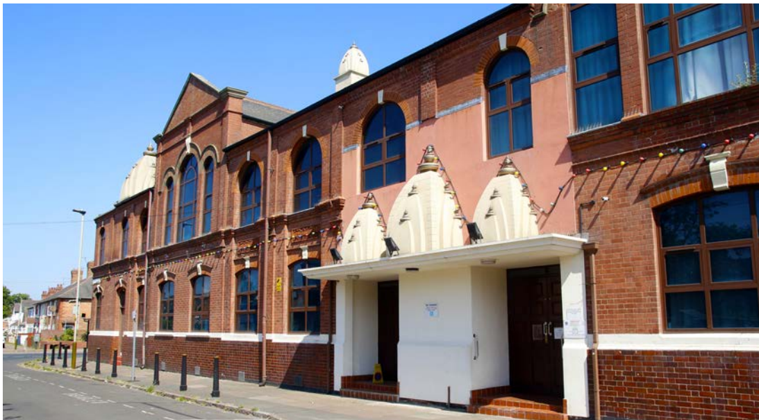
Fig. 23 - The Shree Sanatan Mandir. The façade on Weymouth Street.
