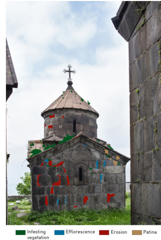
Fig. 7 - Monastery of Haghpat: state on conservation in May 2015 (on left) and identification of degradation form (on right).
