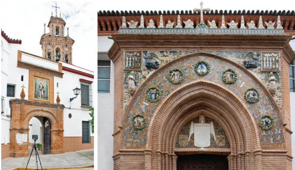
Fig. 2 - Monastery of Santa Paula Seville (Spain): (left) Laser scanner recording of the main entrance brick doorway to the landscaped atrium and (right) detail of the Niculoso Pisano Portal.
