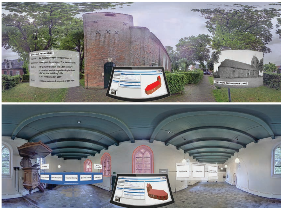
Fig. 8 - The Asset Management tool (DEMO RE Suite) used for on-site condition assessment of the Saint Nicholas Chapel in Obergum, the Netherlands, and management of assets with embedded BIM software.
