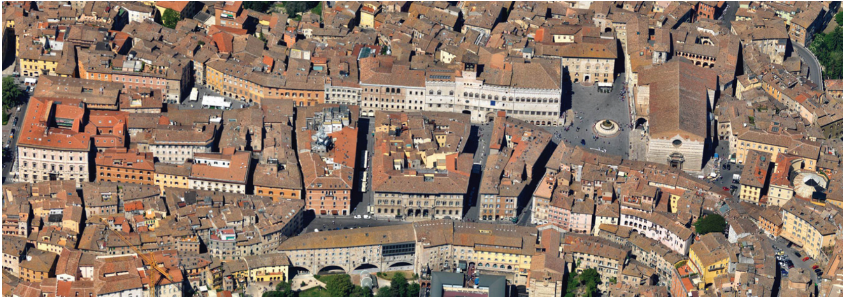
Fig.1 Perugia, aerial view of the acropolis
